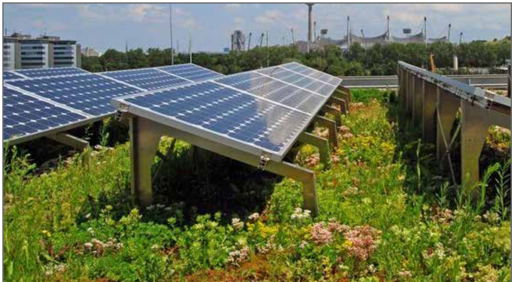
Living roof and solar pv panels
